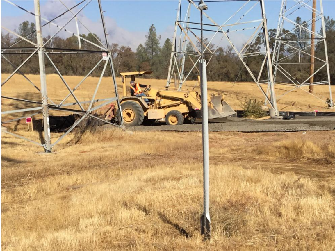
Photo 3: Compaction observed during winterization at Landing Zone 0/1 for future reconductoring work at the Palermo Substation.
