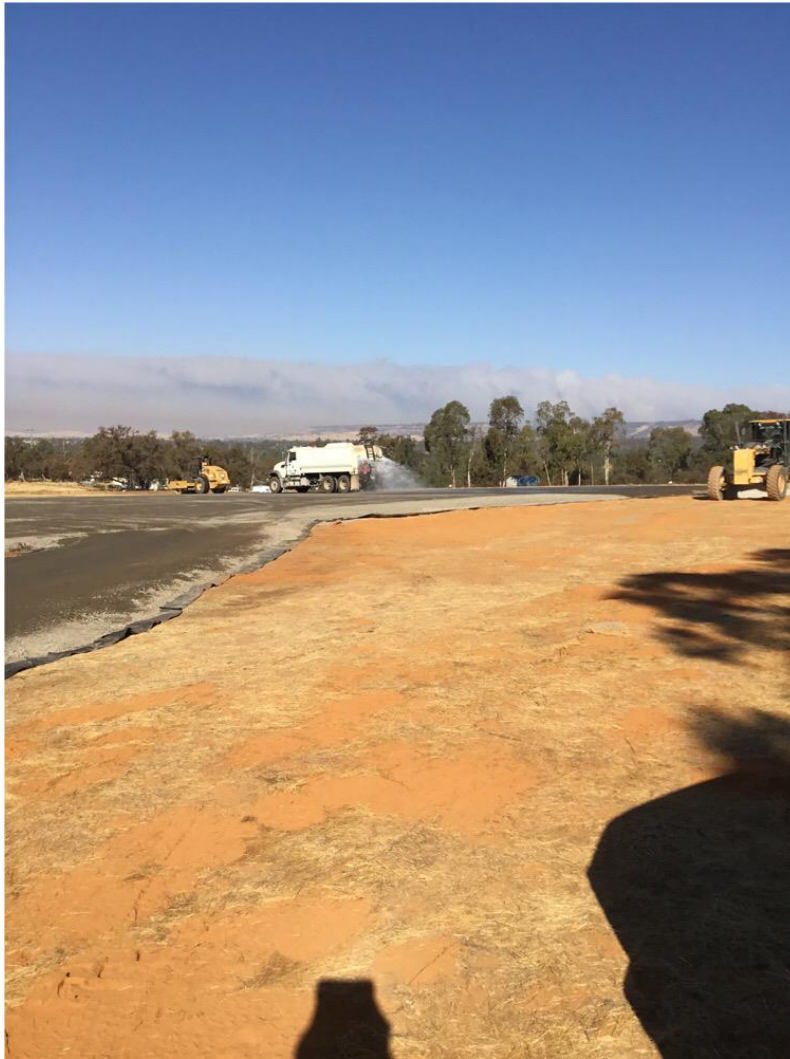
Photo 5: Water truck observed to be running regularly, to control fugitive dust in accordance with APM-AQ-2, during winterization activities at Landing Zone 0/1.
