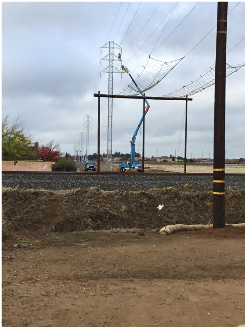
Photo 1: Crews removing transmission line stringing rollers at structure 0/6.
